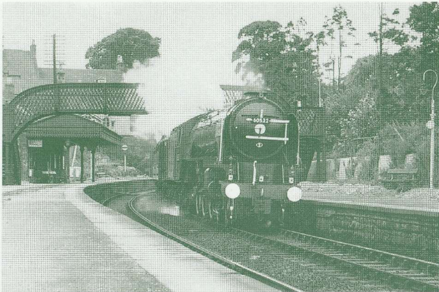
'Blue Peter' July 1966. Note gas pipes removal on platform.
